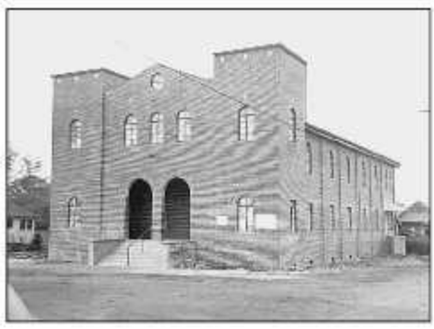
26.a New Bethlehem Baptist Church 1730 11th Ave. N., Bessemer
