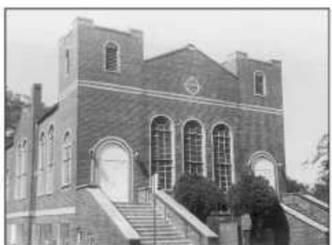
50.a South Elyton Baptist Church 102 1st St. S., Southside
